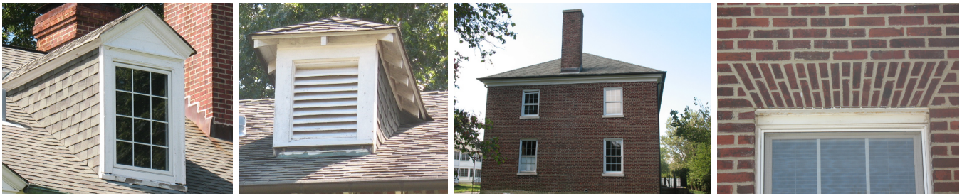
Left to right: Pedimented Dormer, Hipped Dormer, Internal Chimney, Jack Lintel
