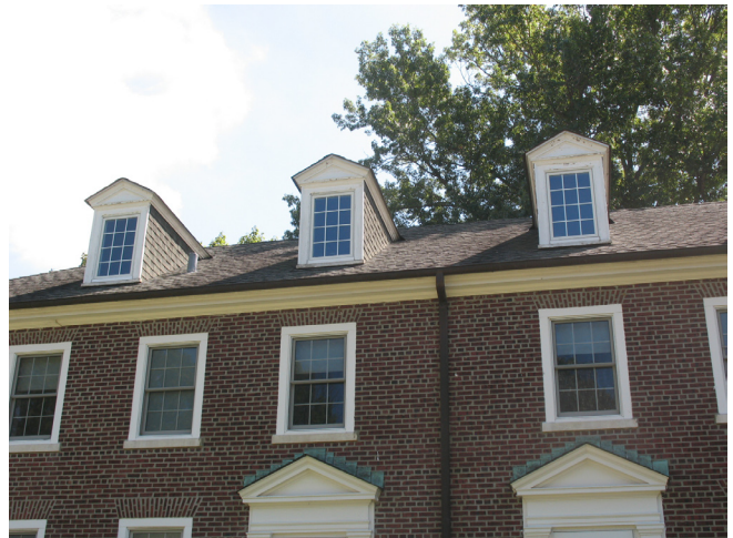
Top: Inappropriate removal of mutins Right: Appropriate replacement of mutins
