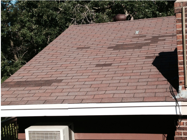
Top: Appropriate asphalt shingle roofing Left: Inappropriate mismatched shingle colors
